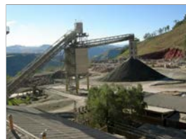
Clinker Production Line
