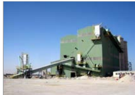
National Cement Plant
