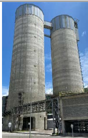
Cement -14.000 Tn single chamber Rio Claro (Colombia) Ecocementos S.A.S.
