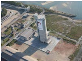
Cement - 18.000 m 3 (6 Chambers) Los Barrios (Cádiz, Spain) Holcim
