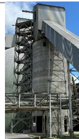
Clinker -1.500 Tn Rio Claro (Colombia) Ecocementos S.A.S.
