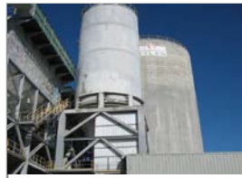
Cement - 1.500 Tn Najayo (Dominican Rep.) Holcim
