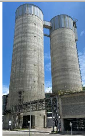
Cement -14.000 Tn 3 - chamber Rio Claro (Colombia) Ecocementos S.A.S.
